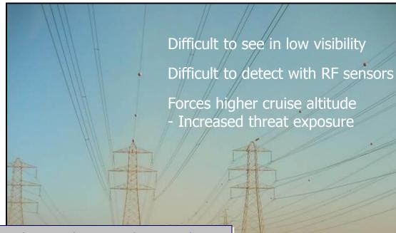
Wire strikes are the number one threat to low flying aircraft during training operations. During armed conflict, low altitude obstacles (wires, towers, etc.) are the number two threat to low level operations, preceded only by small arms and air defense systems.
